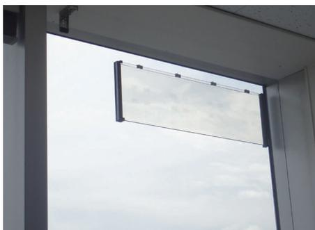
Glass antenna attached to an existing window
