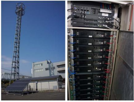
Solar panel and base station (left photo) and green electricity controller (top shelf) and high-capacity, rechargeable battery.
